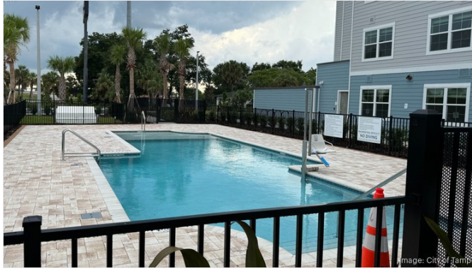
The complex will include a swimming pool, outdoor playground clubhouse area with a meeting room and a fitness center.
